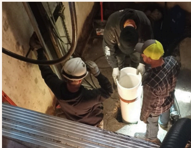
Rock and stones discovered at the bottom, block the new liner from being positioned fully at the bottom (within three feet of jack hole)
