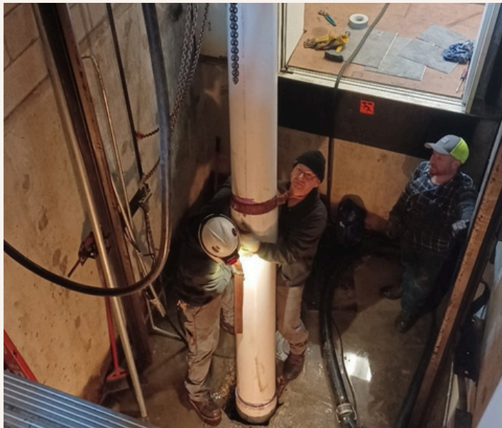
Attempting to install the plastic pipe jack liner
