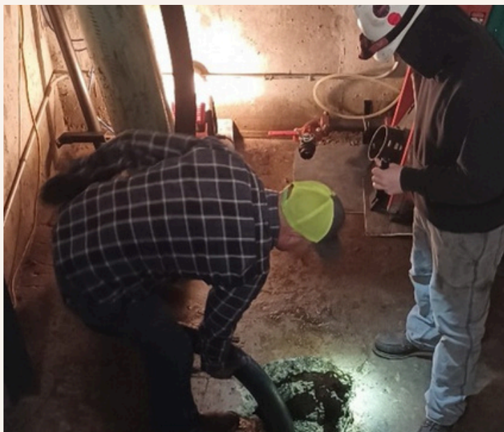
Vacuuming debris from the jack hole
